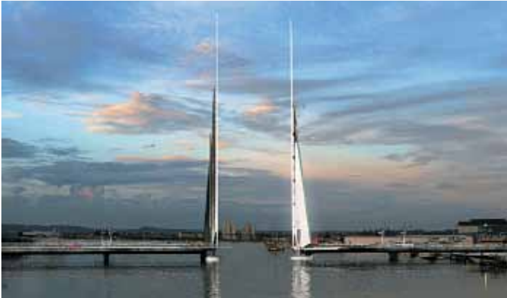
← Twin Sails Bridge now under construction
